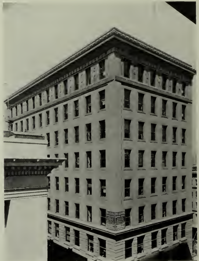
THE SECURITY BUILDING. Howard & Galloway, Architects.
